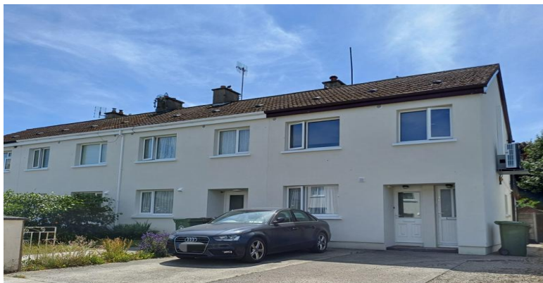
Energy Retrofit works completed at Seamount Drive Kilcoole 2025.
